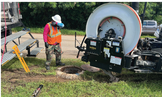
Wastewater Grout CCTV Inspection Truck
